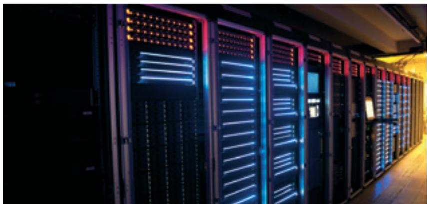
power entering a data centre by the power used to run the infrastructure within it. PUE is therefore expressed as a ratio, with overall efficiency improving as the quotient decreases toward 1. From an average figure of over 2.5 only a couple of years or so ago, PUE is now typically below 2 with new data centres achieving 1.5 or lower. Most of this improvement is the net result of better design based on experience, innovation and energy management advances.
