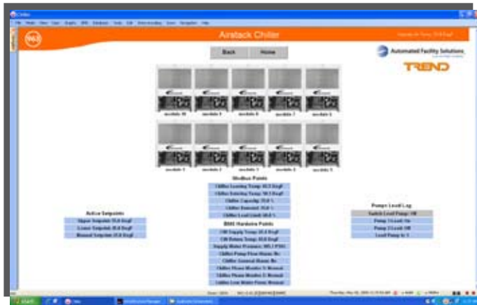
A graphic of the Airstack chiller gives Qualcomm technicians comprehensive at-a-glance information about both the equipment and the environment.
