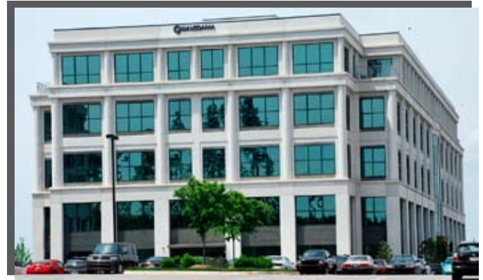
The Qualcomm data center in Raleigh houses a new Trend building management system that integrated multiple systems and now monitors more than a thousand control points.
